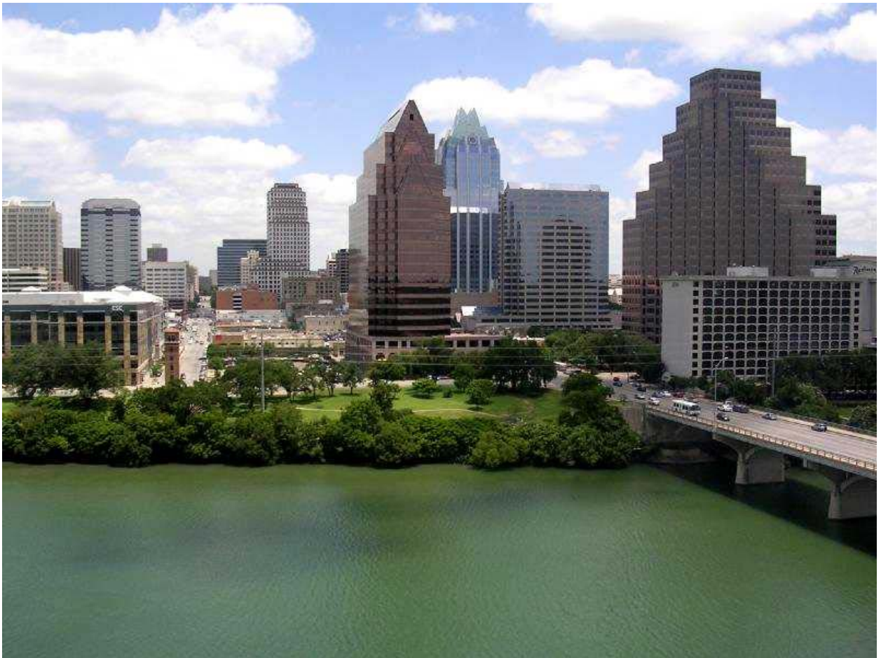
Congress Avenue Bridge, City of Austin
